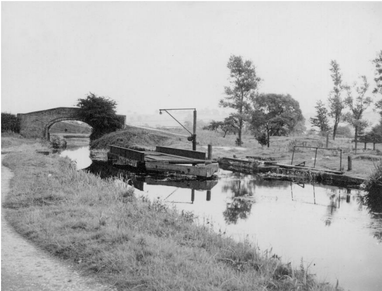
Apparently the crane (left) was used to lift China/Cornish Stone out of the boats, and to lift larger rocks directly into the railway trucks.
