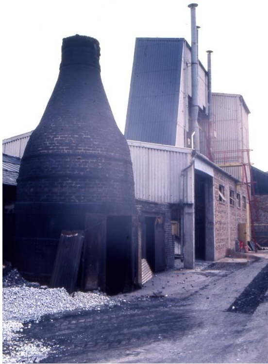
Later comparison to calcining flint - from intermittent kiln to a continuous vertical gas fired kiln
