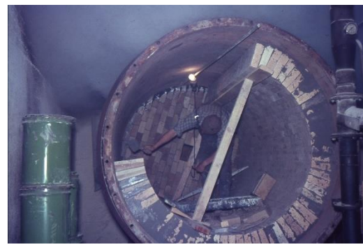
Furnace re-line with specialised bricks.
