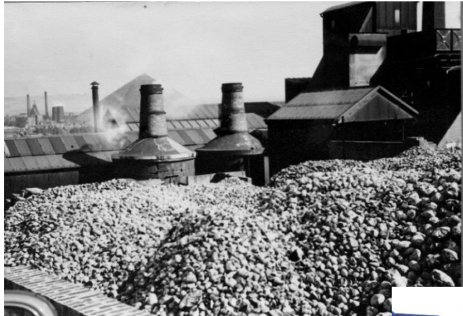
Left: Flint pebbles stock-piled after delivery by canal (c. 1950). Calcine kilns, middle ground.
