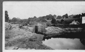
HERCULES MILL after floods from STANLEY POOL RESERVOIR following cloudburst. July 1927.
