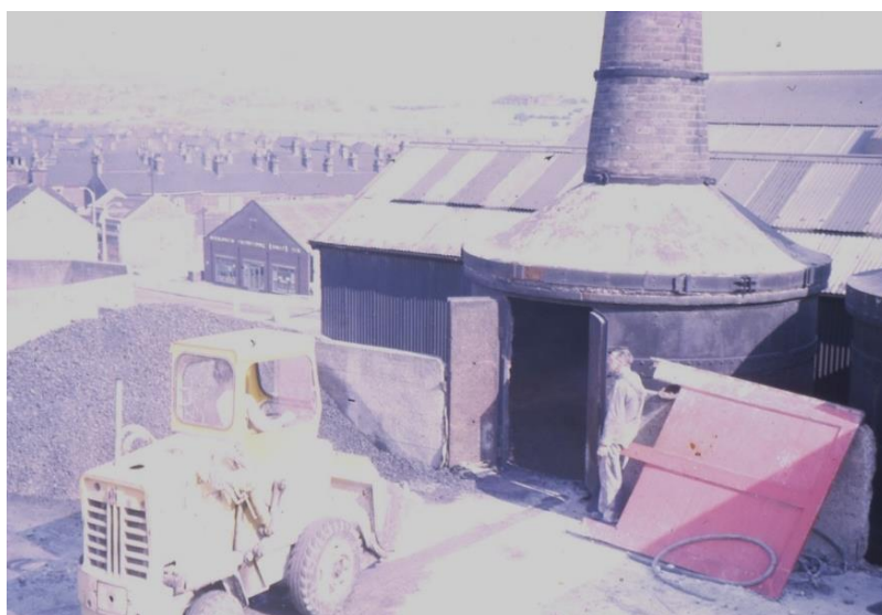
Charging the flint kiln mechanically (c.1965) instead of the old method of men with wheel-barrows. Note the man by the door who shovelled in layers of coke.
