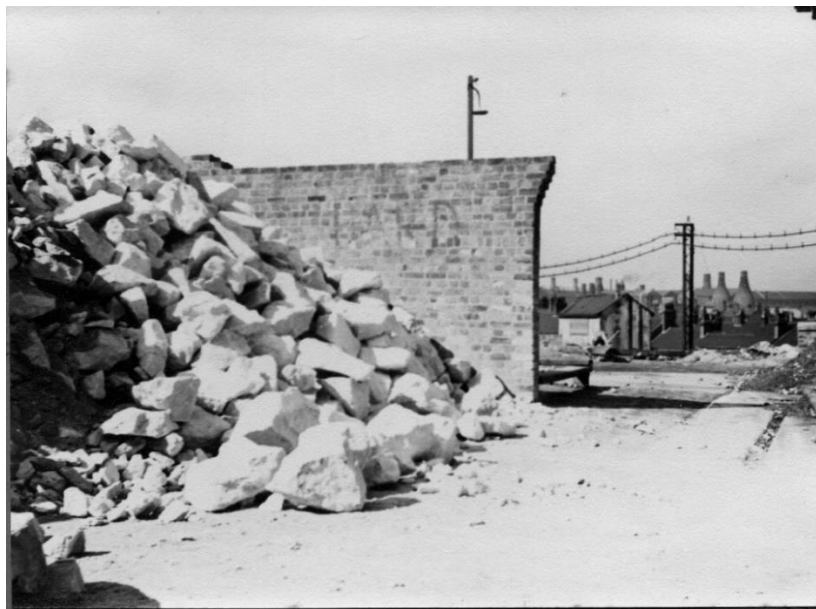
Stock-pile of Stone at Joiners Square Works
